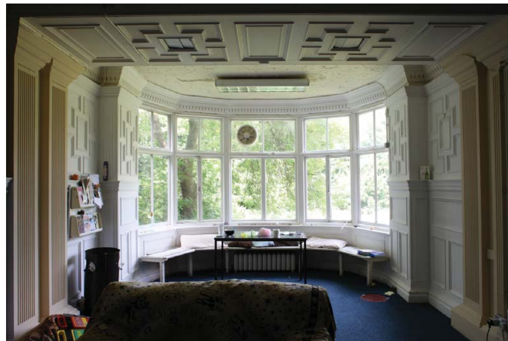
Ceiling and wall panelling/cornices
