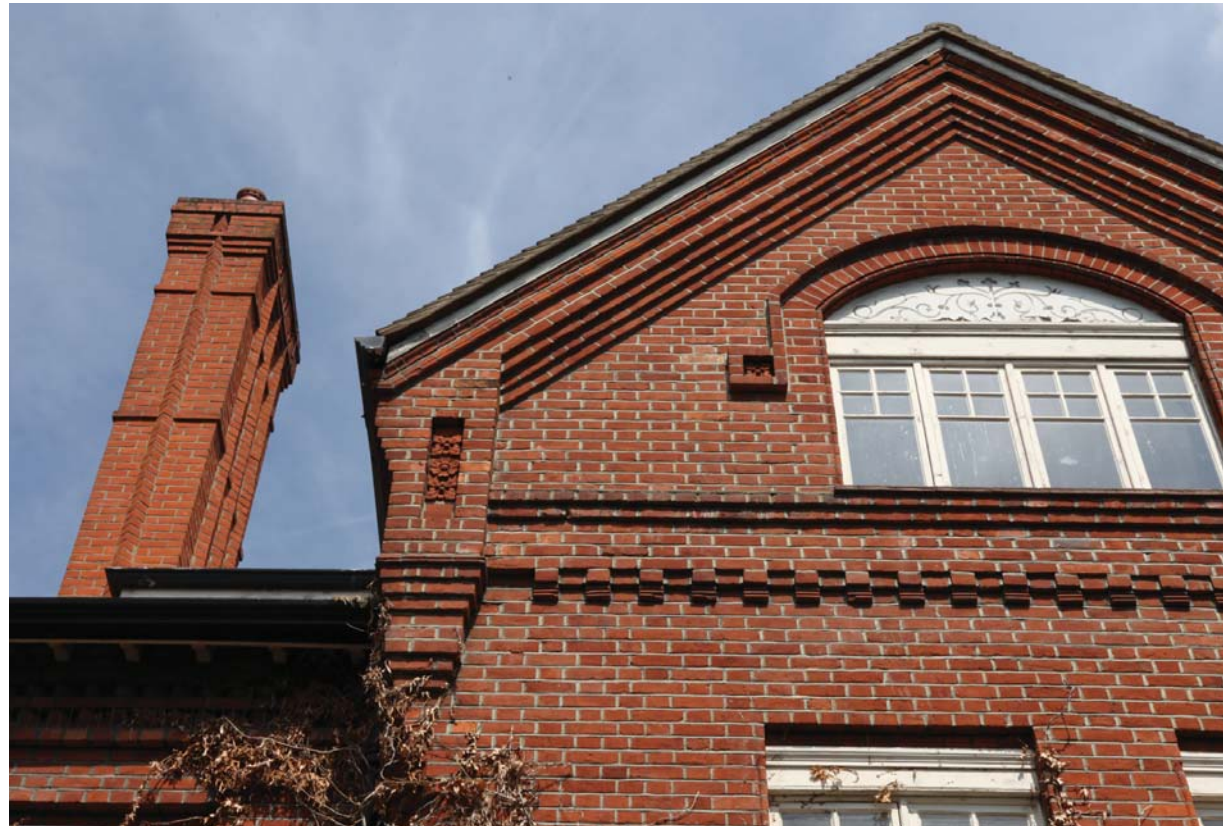
Brick cornices, arched windows, decorative eaves, gabled end roof, arches above windows
