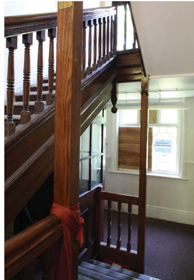
Main staircase with timber balusters
