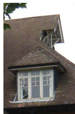
Irregular roof line, dormer windows
