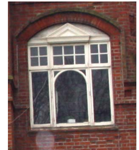
Pointed arched window
