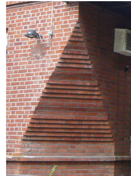
Flemish brick coursing
