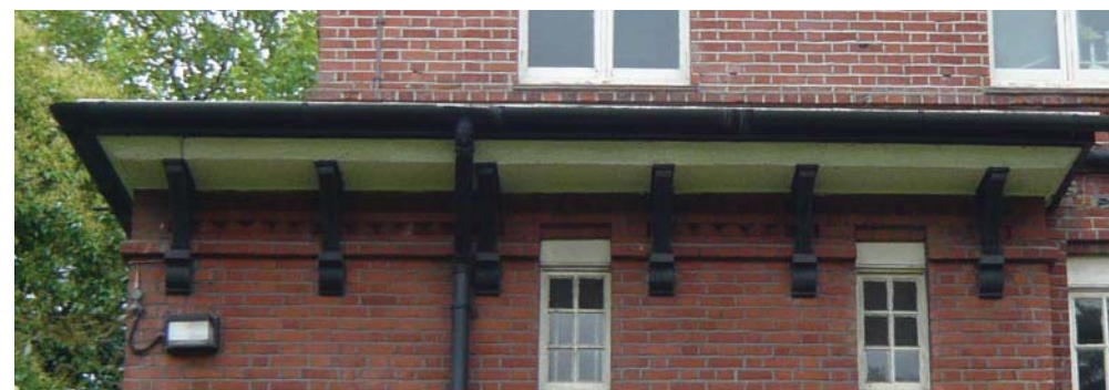
Decorative brackets beneath eaves
