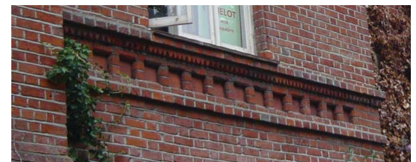
Decorative brick reveals and sweeps
